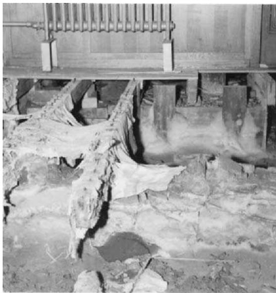
**Fig 2.7** Severe attack of dry-rot exposed (with kind permission of Rentokil)
