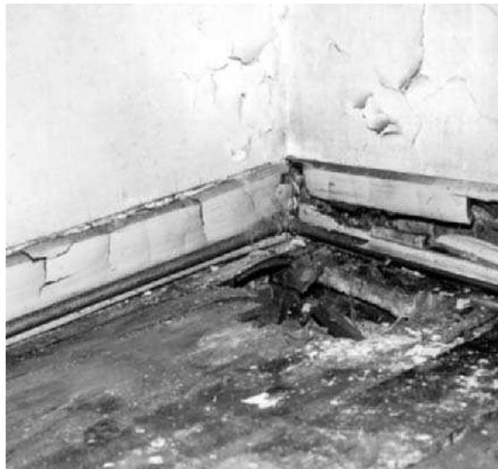
**Fig 2.6** Surface effect of a dry-rot attack (with kind permission of Rentokil)
