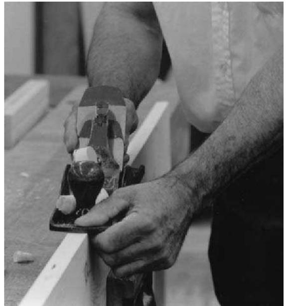
**Fig 5.41** Edging – planing the edge of a piece of timber held in a bench vice with finished face positioned towards the operative – four fingers acts only as a guide to centralise the plane during the operation – not as a fence
